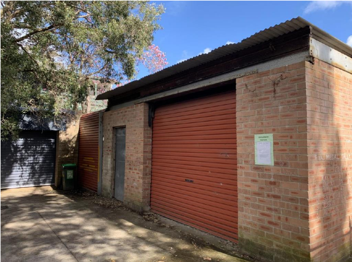
Figure 3: Existing garage and separate roller door as viewed from Kingsclear Road. It is proposed to demolish the existing structures and construct a laneway structure with ground floor garage with studio above.
