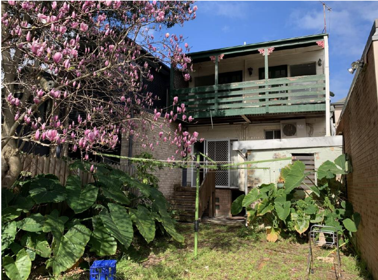
Figure 4: Site viewed from the rear private open space showing a significant magnolia within the rear private open space
